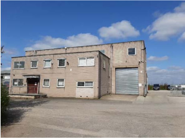
Front elevation of existing building.
